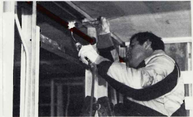
Figure 3: On site brazing.
